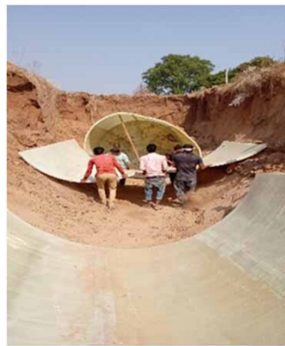
Figure 9 | Assembling GRP panels of the directional tunnel.
