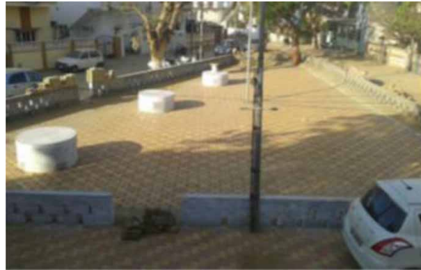
Figure 10 | Groundwater recharge scheme constructed on common ground to deal with flood problems.
