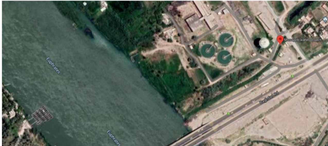
Figure 1 | Al-Mussaib water treatment plant.
