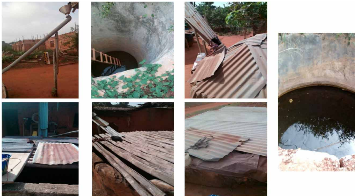
Figure 2 | Rainwater harvesting system in Ekpoma.
