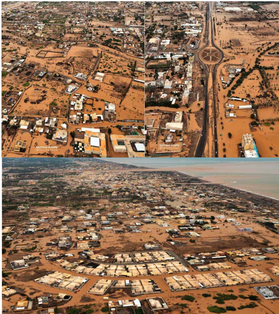
Figure 4 | Different pictures for damage in Al-Khaburah (BBC 2021).
