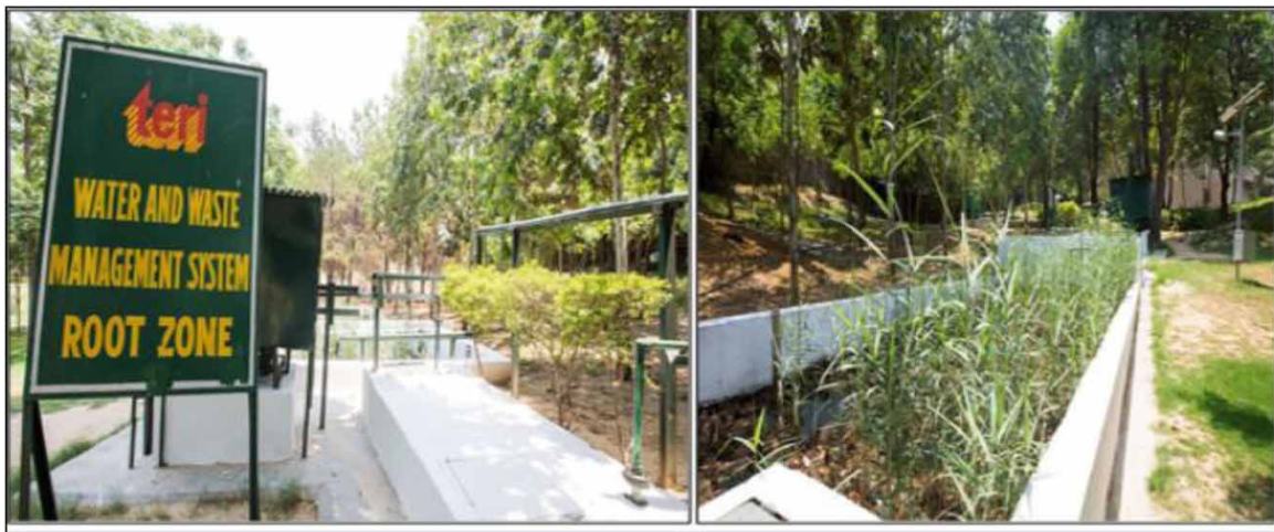
Figure 1 | Photos of TERI's CW-based treatment known as the RZT Plant.
