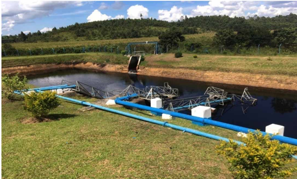
Figure 2 | Intake works, Nyaruzinga water treatment plant.
