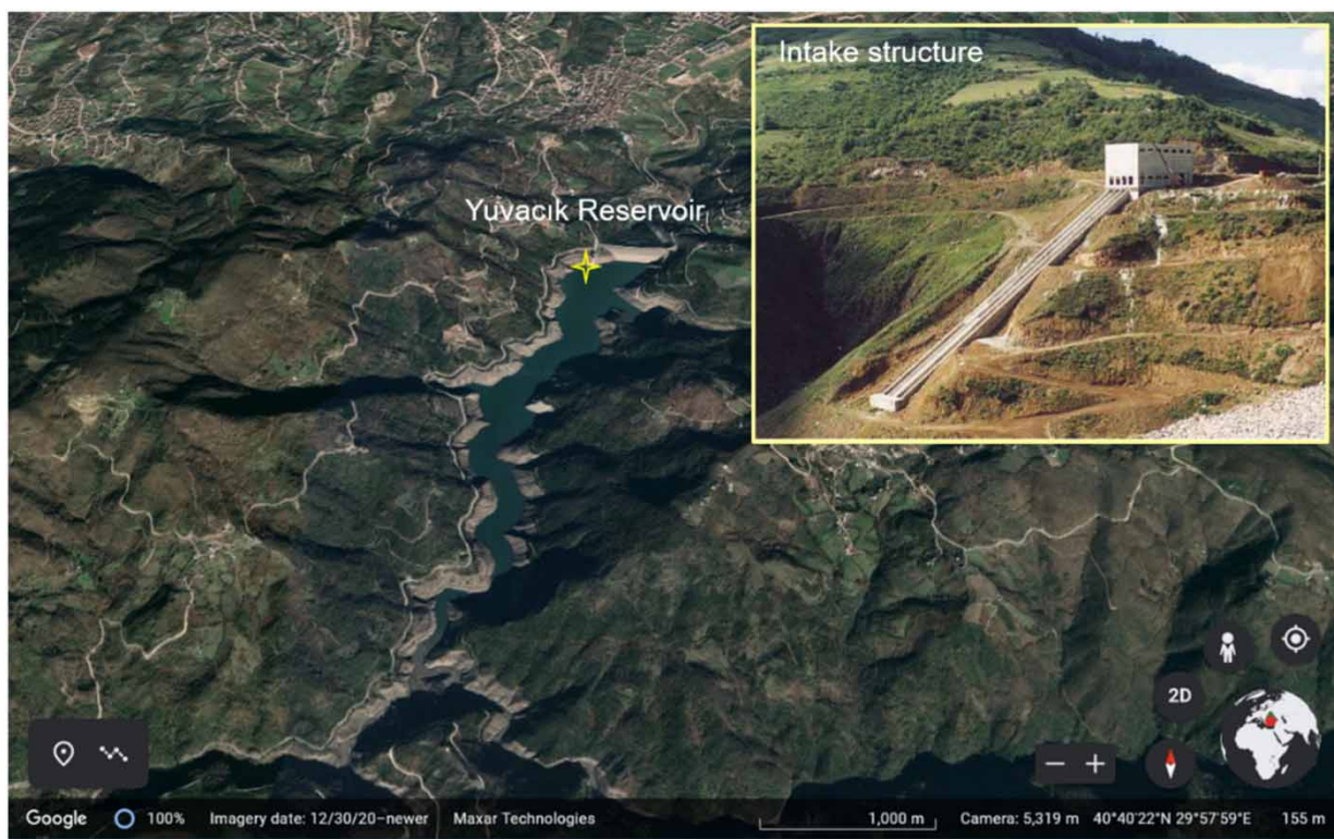
Figure 2 | Satellite image of Yuvacık Reservoir (Google Earth, June 2022) and intake structure at the construction time (İSAŞ 2022).
