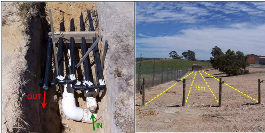
Figure 2 | (a) Construction image of partially buried pipe connections (single PDS) highlighting arrangement necessary to achieve 1.05 km of pipe length in compact spacing; (b) buried PDS from far end (with air purge valves) looking towards entry/exit points.
