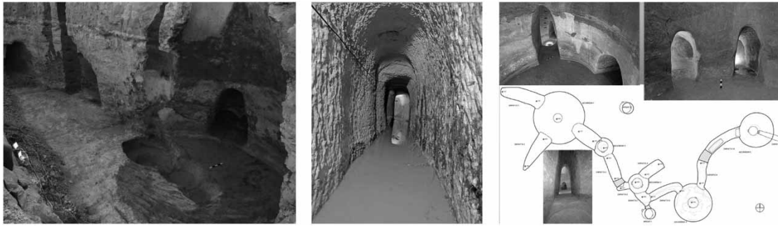
Figure 4 | Piraeus, rainwater harvesting system, multi-chambered rock-cut cisterns, linked with wells through vaulted tunnels ( https://ocw.aoc.ntua.gr/courses/CIVIL100 ).
