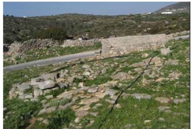
Figure 7 | Byzantine-era cisterns in Amorgos: a small, vaulted one with an orifice (Mays et al. 2013) and another flask-shaped on the left along with the partially paved runoff surface (G. Antoniou).
