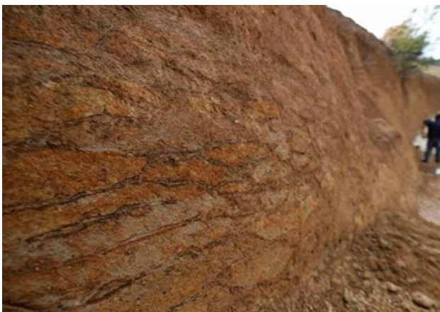
Figure 1 | Liangsu culture dam in which grass and clay are interlining.
