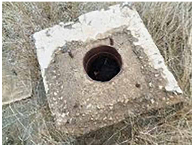
Figure 5 | Abandoned borehole; main hole destroyed.
