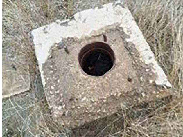
**Figure 5** | Abandoned borehole; main hole destroyed.
