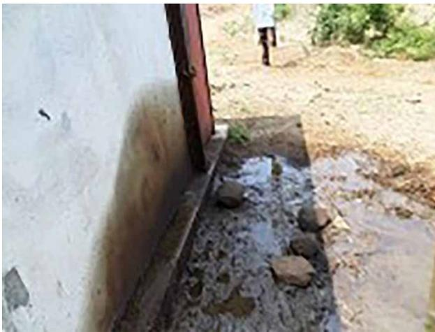
**Figure 4** | Stagnant water around borehole.
