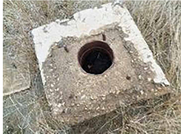
Figure 5 | Abandoned borehole; main hole destroyed.
