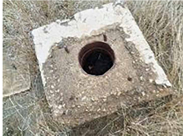
Figure 5 | Abandoned borehole; main hole destroyed.
