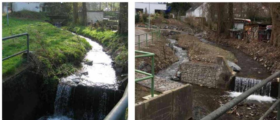
**Figure 3** | Restoration of river continuity at an existing drop structure (left) by bypassing it via a new water course (right).
