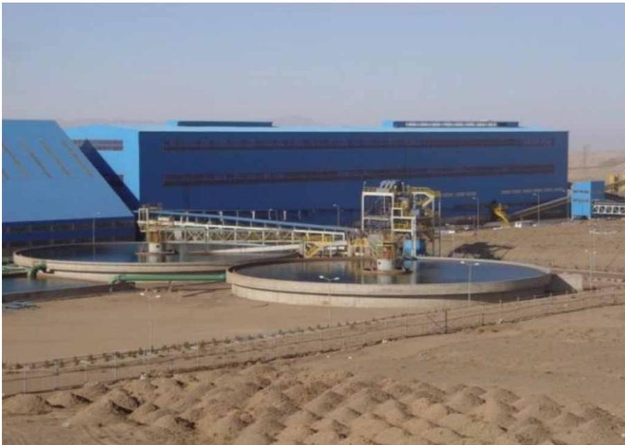
Figure 2 | Concentrator and thickeners.
