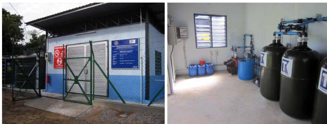
Figure 2 | Small-scale water treatment plant (left) and the conventional sand/media filtration system.
