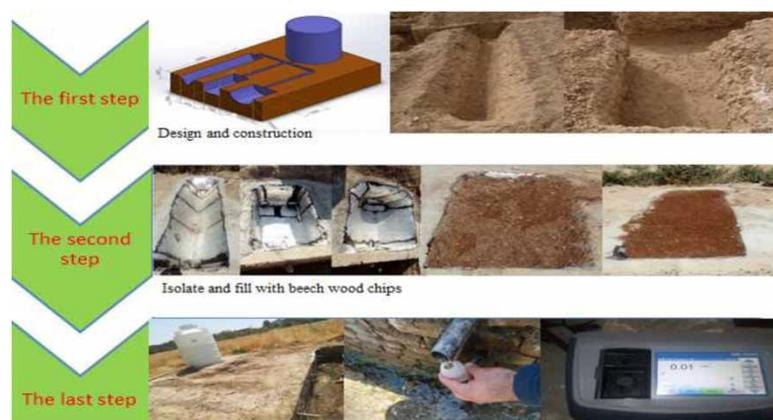
**Figure 1** | Flowchart: In the first stage, bioreactors were designed by Tri-Di max software and the necessary excavation was performed. In the second stage, the bioreactors were made of brick and cement, insulated with a waterproof membrane, and filled with beech woodchips. In the last step, the bioreactors were covered with plastic and by adding the necessary materials to the tank, the experiment was started, sampling was performed and the data were analyzed.
