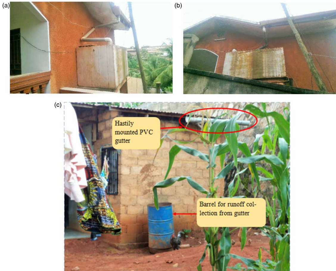
Figure 5 | Well-elaborated and rudimentary roof-harvested rainwater systems in the Mvog-Betsi neighbourhood.
