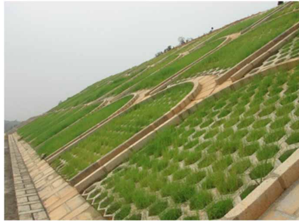
Figure 6 | Application effect of ecological slope protection.
