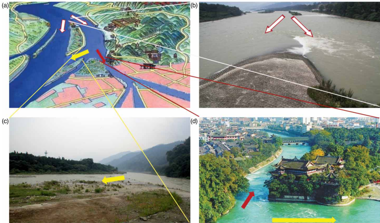
Figure 4 | Dujiangyan Irrigation Project. (a) Schedule for Dujiangyan Irrigation project; (b) the water-diversion rule of Fish-mouth; (c) Spillway of the Flying Sand Fence; (d) Gate of the Bottle-Neck Channel.
