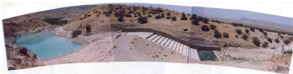
Figure 3 | Tang Khon earthen dam in Bushehr province, Iran and its stepped spillway.
