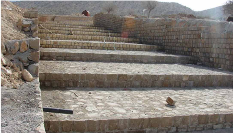
Figure 4 | A stepped chute from Moradabad earthen dam in Firoozabad city, Iran.
