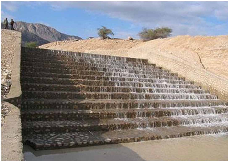
Figure 2 | A stepped chute constructed in Kohkiluyeh city, Iran.
