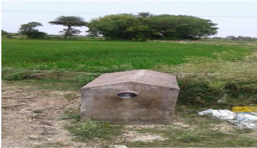
Figure 3 | Water distribution system in Deevanur tank.
