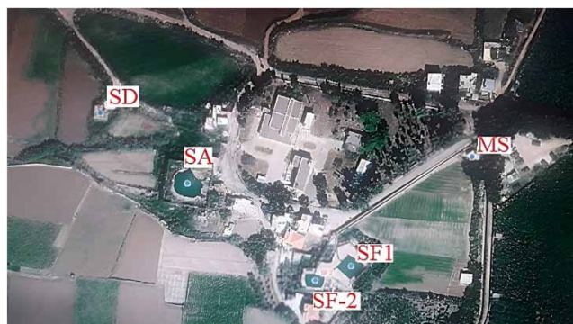
Figure 1 | Ras El-Ain natural ponds and water department.
