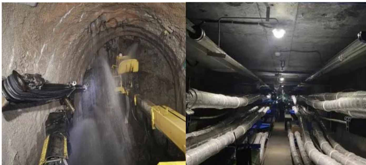
Figure 2 | Tunnel treatment after water disasters.
