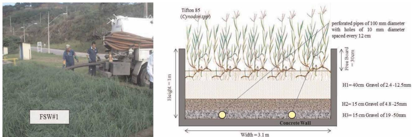
Figure 1 | Full-scale unit receiving sludge and schematic cross section of each unit.
