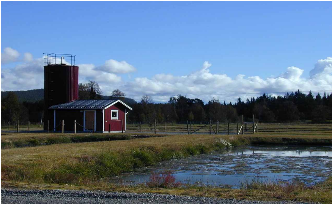
Figure 1 | The fellings dam at Hede (pop. 3,000) with dosage station, a pre-settling pond and seven post-settling ponds in the background.
