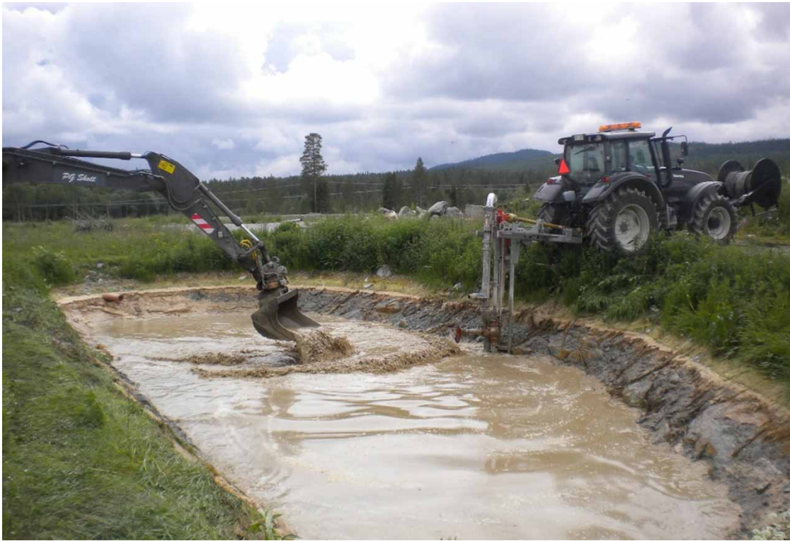
Figure 6 | Sludge emptying by a combination of pumping and excavation.
