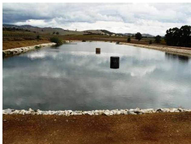
**Figure 1** | Facultative waste stabilisation pond at Lyndoch, SA, wastewater treatment plant.
