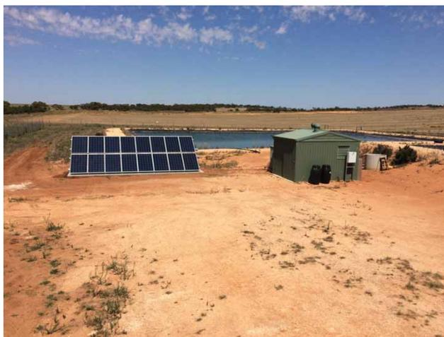
**Figure 4** | The 5.3 kW h<sup>-1</sup> solar voltaic cells installed at the Kingston on Murray, SA, wastewater treatment plant.
