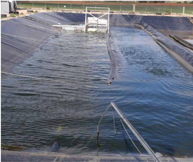
**Figure 2** | High rate algal pond at the Kingston on Murray, SA, wastewater treatment plant.
