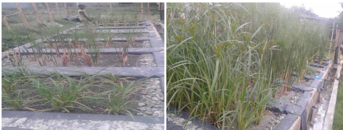
Figure 2 | Picture of the pilot-scaleSSF wetlands to treat hospital wastewater.
