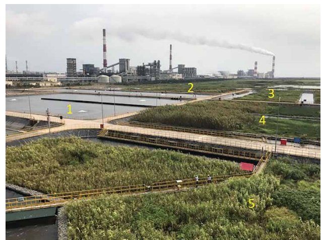
Figure 4 | Hybrid pond – wetland system for Formosa Steel plant wastewater polishing treatment, Vietnam (design flow 36,000 m 3 /day, total area 10 ha). (1) Waste stabilization pond cells; (2) subsurface flow constructed wetland cell CW1; (3) subsurface flow constructed wetland cell CW2; (4) subsurface flow constructed wetland cell CW3; (5) free water surface flow constructed wetland cell CW4.
