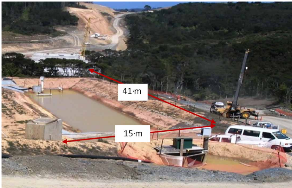
Figure 2 | View of the Alport B2 field pond.
