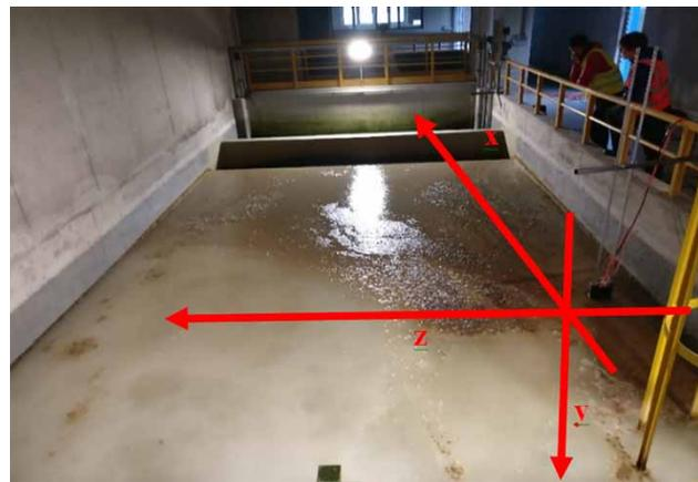
**Figure 4** | Schematic of the measurement campaign with the directions at the DAF utility.
