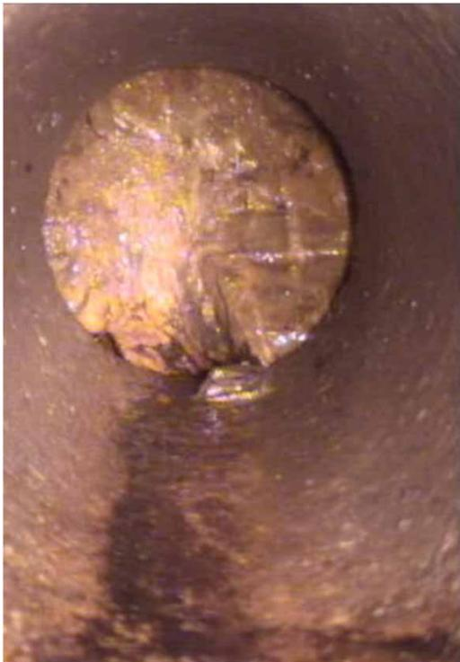
**Figure 4** | Hydraulic restriction (blockage) failure along Henry Street, downtown Port of Spain, caused by the solidification of FOG; it caused an SSO, needing an emergency intervention to be cleared (still from CCTV footage WASA).
