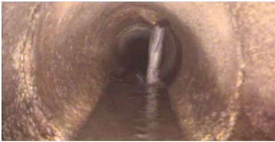
Figure 6 | CCTV still showing excessive infiltration in the sewer line along Park Street, Port-of-Spain (still from CCTV footage WASA). It eventually caused an SSO, leading to an emergency intervention as well.
