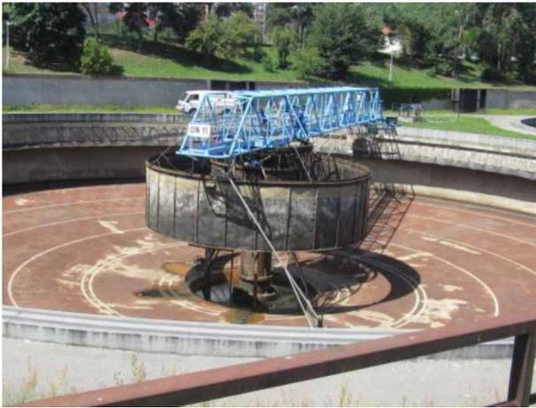
**Figure 2** | Secondary clarifier of Prague Central WWTP from 1997. Horizontal flocculation zone, spiral blade sludge scraper, Stamford baffles; sidewall depth 4.4 m.
