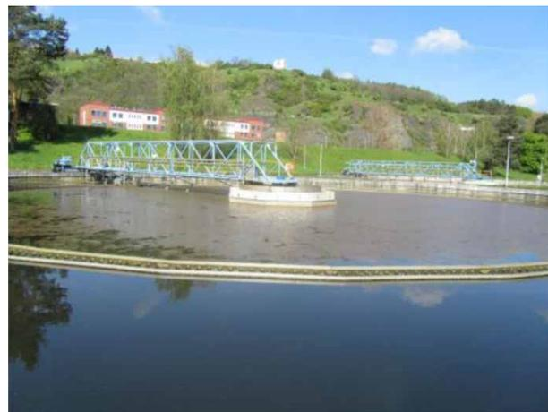
**Figure 1** | Secondary clarifier of Prague Central WWTP from the 1960s. Simple energy dissipating well in the center, in-board effluent launder (scum baffles were added later), no surface skimming, sidewall depth 2.5 m.
