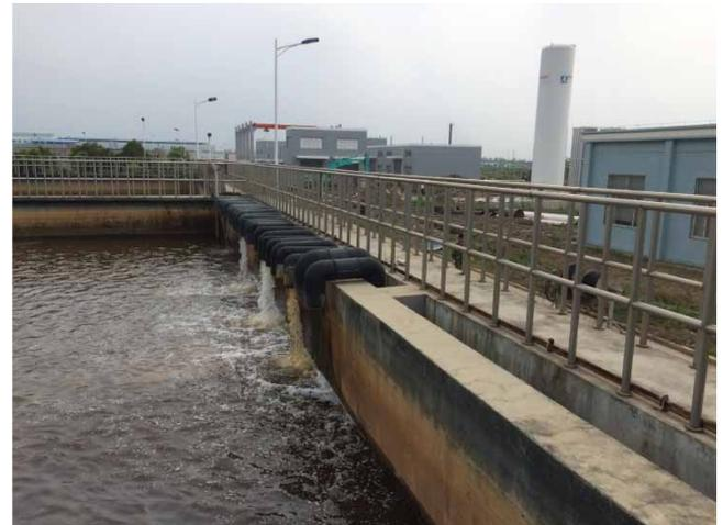
**Figure 2** | Photo of the common wastewater collection pool at the centralized WWTP, with the tailpipes of individual wastewater transmission pipelines from different companies.
